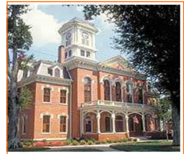
The Walton County Courthouse is a Greek Revival style building built in 1845. It is at the heart of Monroe's historic district.
